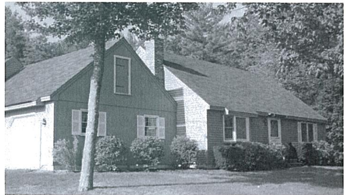
Photograph 2: Nice House Over Icky Crawlspace —This house with the crawlspace problem is in Washington, DC
