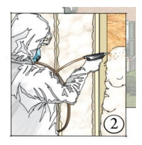
Spec blown-in or sprayed-in insulation products to improve energy and air-leakage performance.
