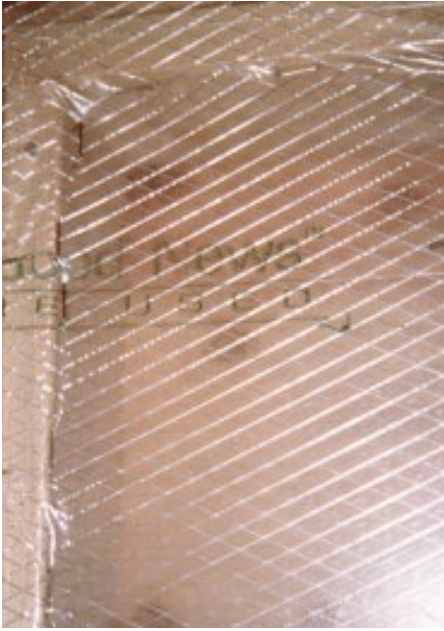
Figure 8. Most dense-pack cellulose systems require the installation of a reinforced polyethylene air barrier. Stapling the poly on the side rather than the edge of the studs helps keep the poly from bulging when the cellulose is blown in place.
