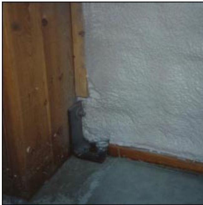
Details that are difficult with sheets and caulks are little challenge for Spray Foam.
