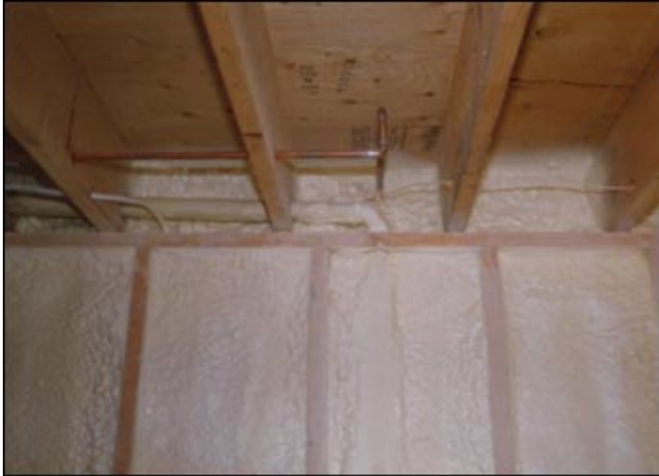
Rim Joists – above foundations and between floors are vapor retarded, insulated and air barriered with complete moisture control in a single application of the closed cell spray polyurethane.
