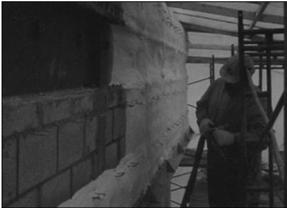
Courtesy: CHEM-THANE, Concord Ontario, CA Ease of sustaining air-barrier continuity in complex situations.
