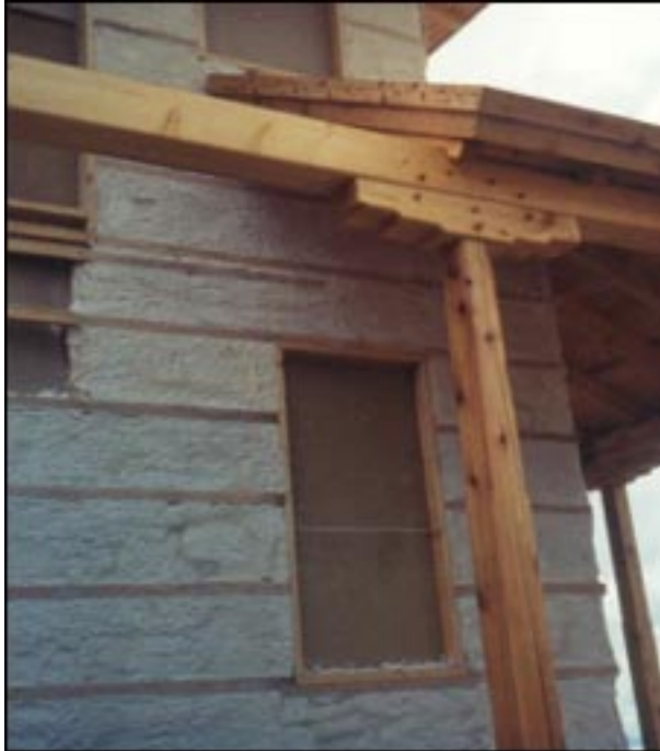
Timber frame application before siding.
