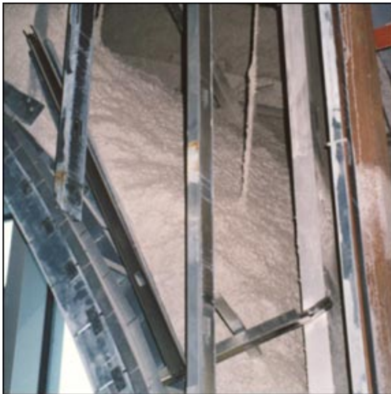
Monona Terrace Convention Center, Madison WI. Complex arch shapes using CORBOND and Thermal Barrier.
