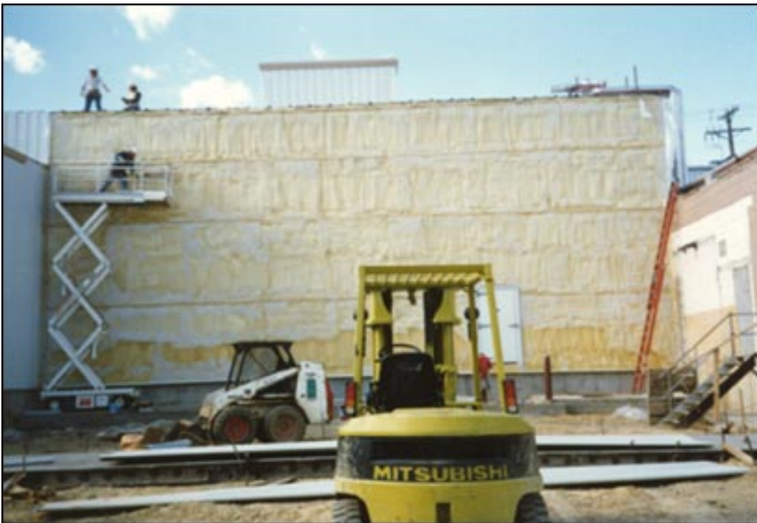
...giant cold storage have used closed cell polyurethane SIP's and spray in place for that long as well.
