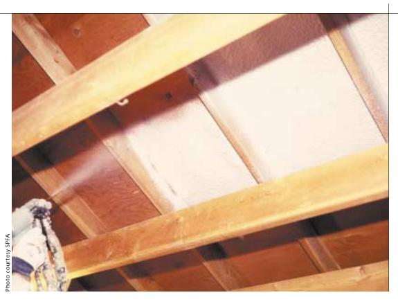
Low-density polyurethane foam sprayed in between floor joists serves triple duty as insulation, air barrier, and sound control device.
