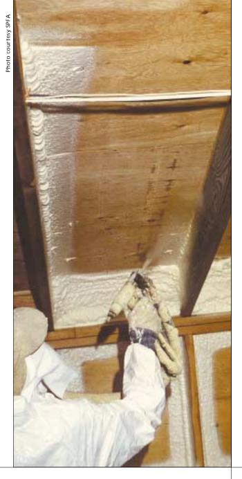
SPF reduces thermal bridges in the building envelope, thereby maintaining more consistent climatic levels as set by building occupants.
