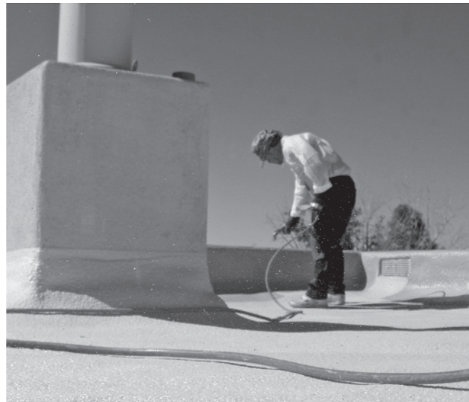
Figure 4. Another option to protect SPF roofing from ultraviolet light is a sprayed-on coating. Most roof coatings last for 10 to 15 years before they need to be renewed. [Photo credit: Thermal Coatings and Insulation]
