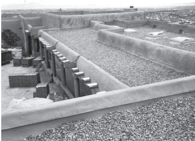
Figure 1. In the Southwest, where traditional architectural styles favor flat roofs, spray polyurethane foam roofing is fairly common. The SPF roofing on this home is covered with aggregate ballast. [Photo credit: North Carolina Foam Industries]
