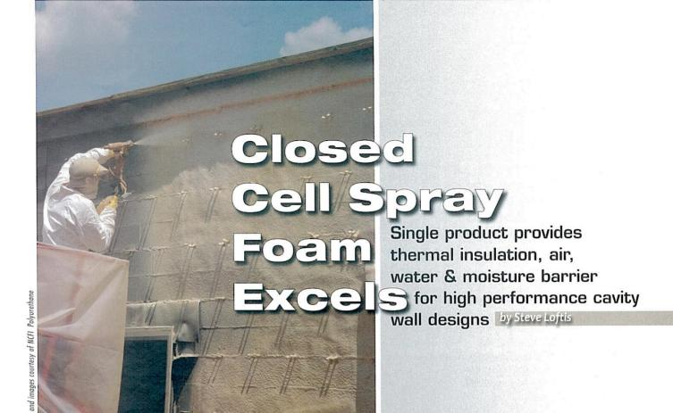
Closed Cell Spray Polyurethane Foam gives full coverage and expands in place, which allows it to air seal construction gaps, plumbing and electrical penetrations, as well as joints of dissimilar materials such as roof deck/wall junctions.
