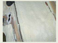
Closed-cell foam was sprayed too thickly into this stud bay and has shrunk away from the framing as a result of exothermic heat build-up. The foam should be removed and replaced.
