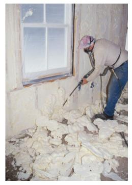
Open-cell foam can be installed in a single pass (above left), but because of its high expansion rate it must typically be trimmed after installation, which produces considerable waste (above). Trimming usually isn't necessary with closed-cell foam, but to avoid excessive exothermic heat, it should be installed in lifts no more than 1½ inches thick (left).
