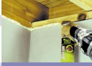
"Before Hurricane Allen blew onto South Padre Island with sustained winds over 125 mph, my company installed a portion of an SPF application to the office section at a lumber yard's post frame construction building. The crew completed one corrugated wall and roof section before the storm hit. We discovered upon our return that the storm carried away all of the metal except where we had applied SPF."
