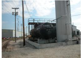
Installer: Martin Gudino and Oscar Espinoza Type of Job: 19,000 gallon Tank Insulation Square footage of Job: 2000 Square feet: sprayed/coated Equipment Used: Gusmer HF-1600 / Gap Pro Guns Number of people needed for the Job: Two man sp Number of days required by the Job: Three Days Special Requirements: Wind Screen and Fall Protection Foam and coatings used: Gaco Western 273 Roof Foam and Gaco Flex A-30
